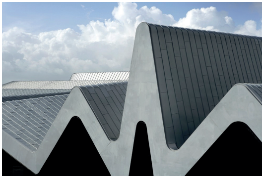
detail of roof
